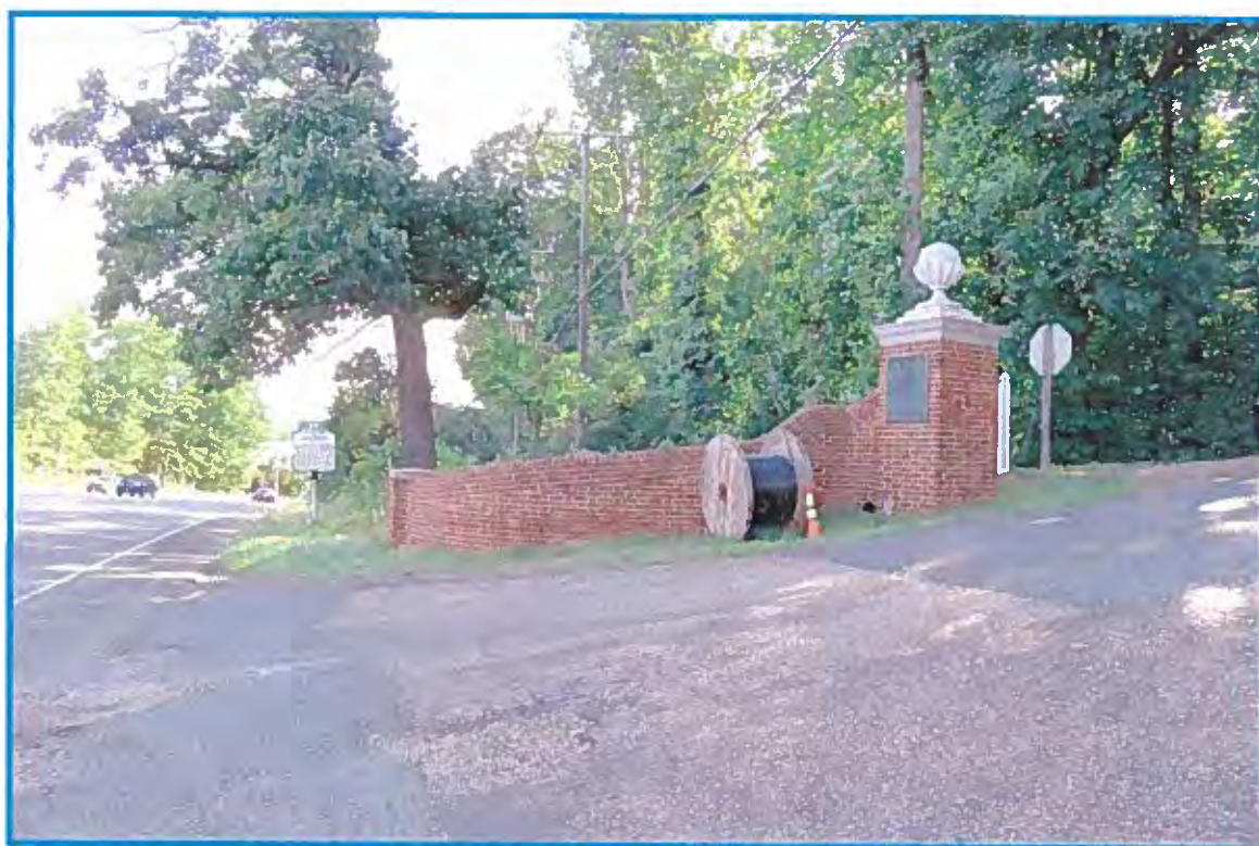
Figure 2. View from entrance to the north.
